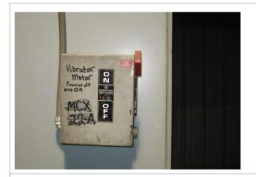
An illustration of labeling on an electrical disconnect identifying the affected equipment.
