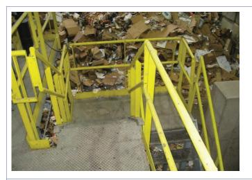
An example of appropriate safety and hand railings on an access stair way.
