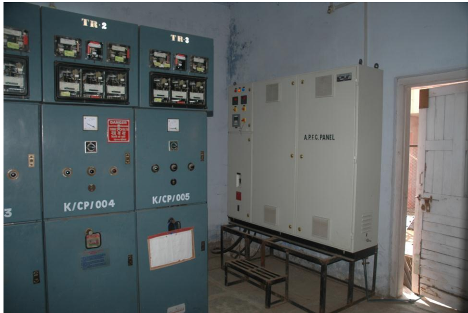
Pic. 8: Thyristor based APFC panel installed at Katargam WW
