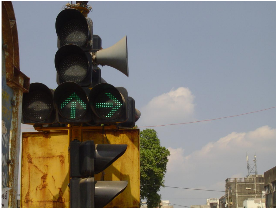
Pic. 2: LED based Traffic Signal panel
