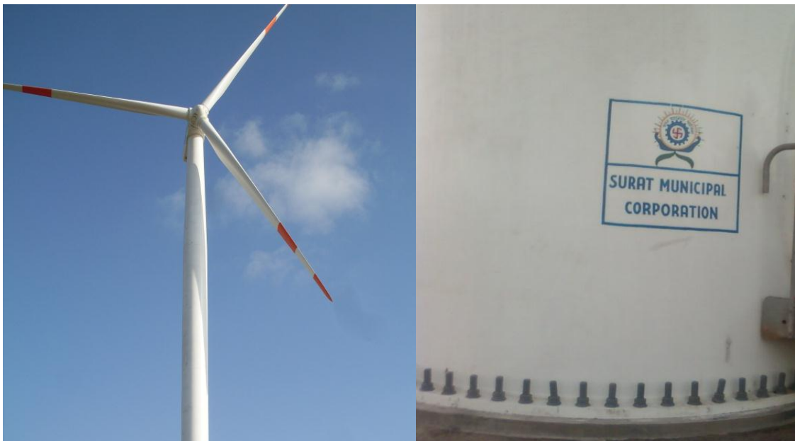
Pic. 3: 1.5 MW Suzlon make Wind Turbine Generator installed at Adodor, Dist: Porbandar
