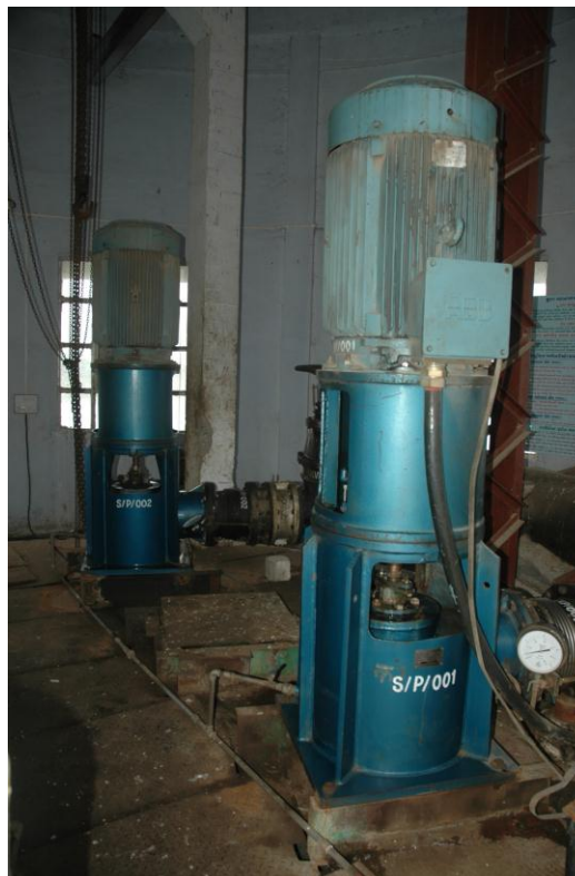
Pic. 7: Replaced pump sets at French Well 1 at Sarthana WW
