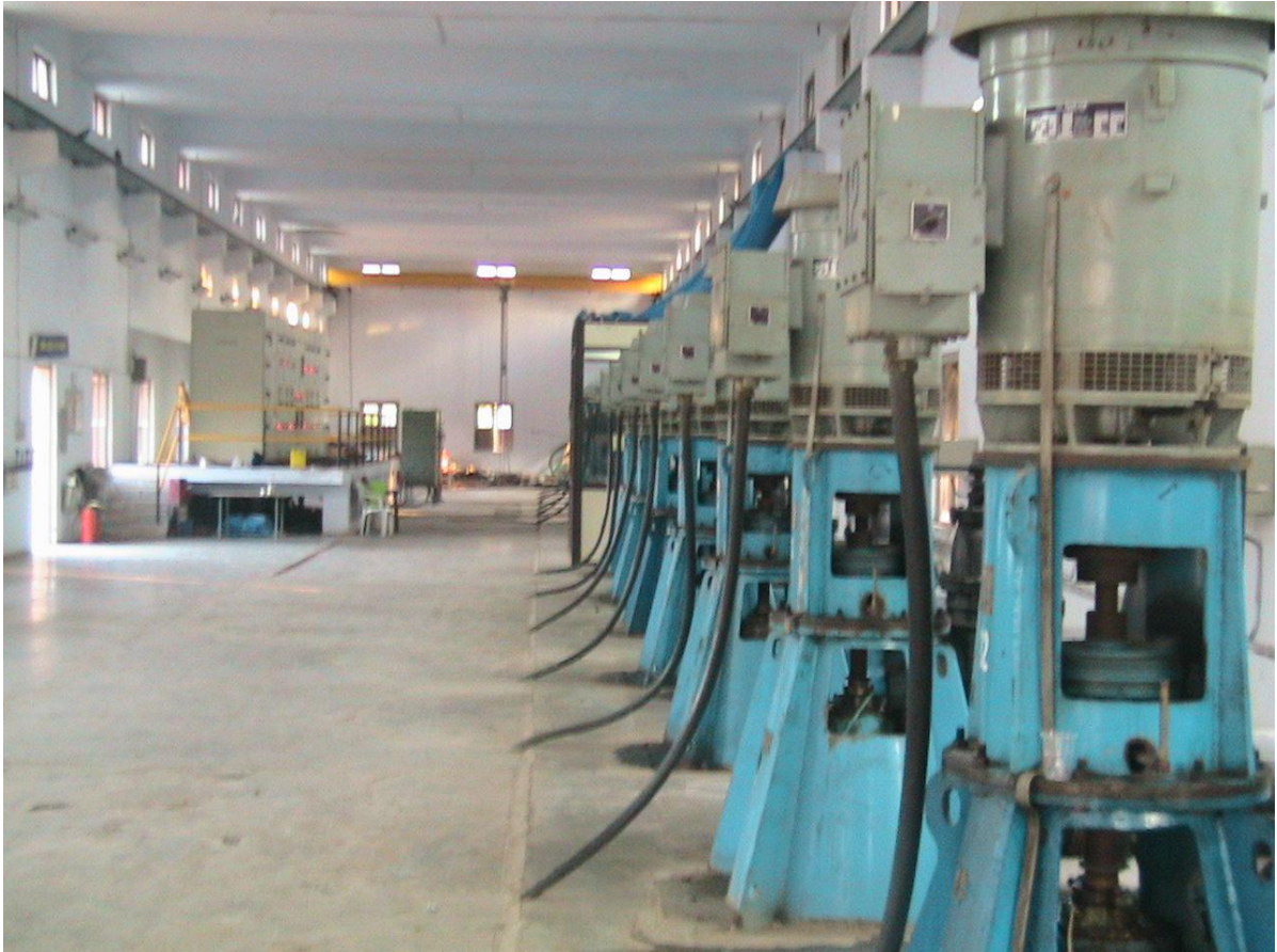
Pic. 1: Replaced pump sets @ Katargam Water Works
