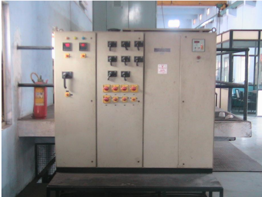
Pic. 4: First Thyristor based APFC panel installed at Dumbhal WDS
