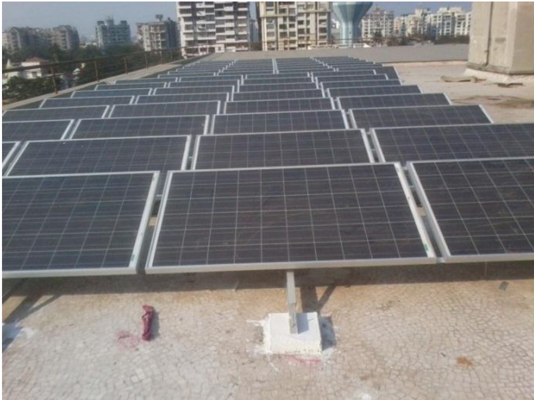
Pic. 10: 100 kWp Solar Photovoltaic Power Plant at Science Centre
