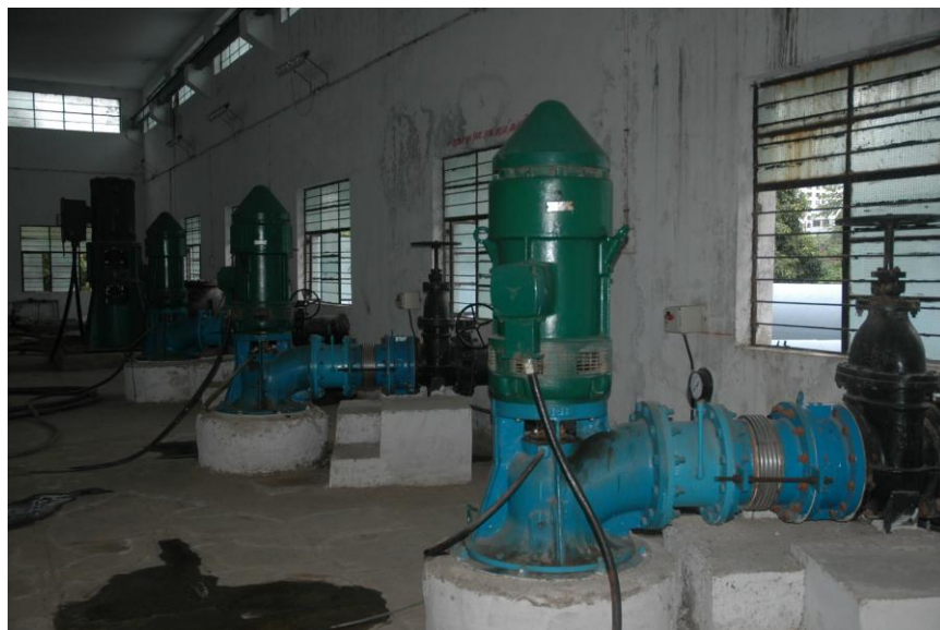
Pic. 5: Replaced pump set at Old Booster House at Sarthana WW
